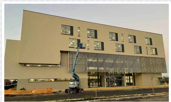
Tlhabane office building (adjacent to the Curro Meridian and opposite the newly constructed mall)
