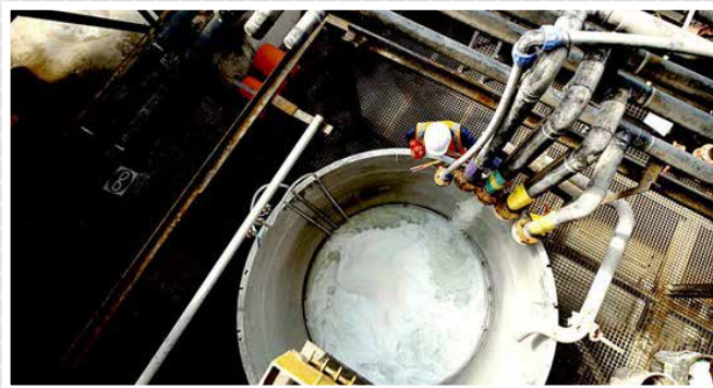
EIHL's liquid fertiliser plant is located in Endicott, South Africa, producing enhanced efficiency liquid fertilisers for the local market
