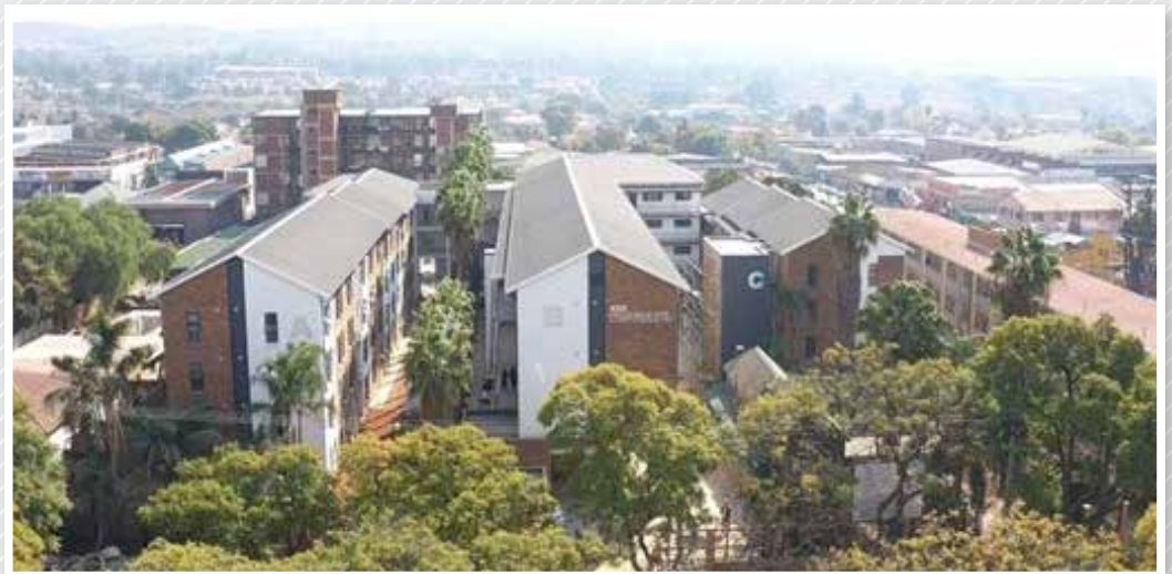
The recently completed Frederick Street student accommodation (ABOVE AND BELOW)
